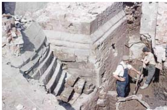
Ruins: 1950s builders dig by the remains of Sheffield Castle's gatehouse, and an augmented reality program shows how the site looked PA
