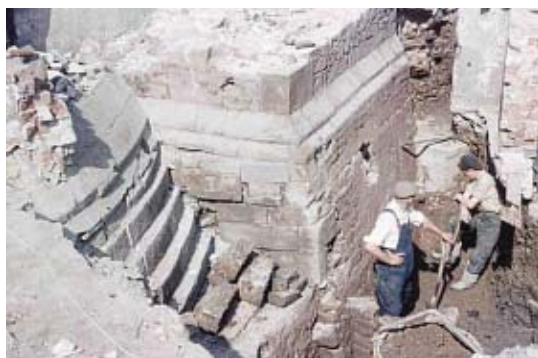
Ruins: 1950s builders dig by the remains of Sheffield Castle's gatehouse, and an augmented reality program shows how the site looked PA
